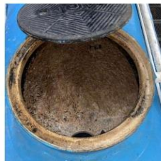
ANAEROBIC FILTER CHAMBER
