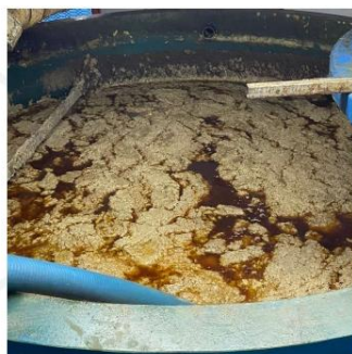
KITCHEN WASTEWATER TANK
